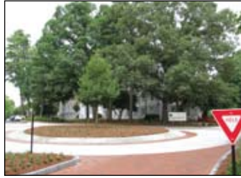
3. Dowman Drive roundabout and streetscapes
