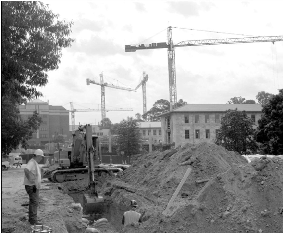
There's little evidence of the parking lot that used to occupy the space next to the Dobbs Center, as the site is being prepared for a new residence hall—the first installment of a planned “freshman village” for the University's first-year students. In the background, the nearest of several cranes rises above the under-construction School of Medicine Administration and Education Building. These two projects in the heart of campus (both due for completion in summer 2007) are two of Emory's higher profile capital projects this summer, but the total list is closer to 20, both large and small.
