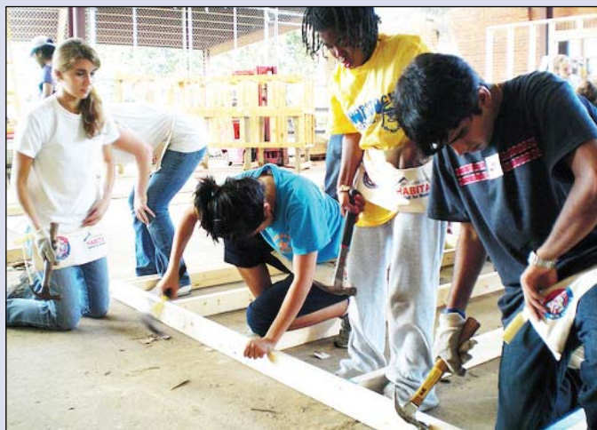
A Habitat for Humanity build in Americus gave students hands-on experience while experiencing Georgia history.
